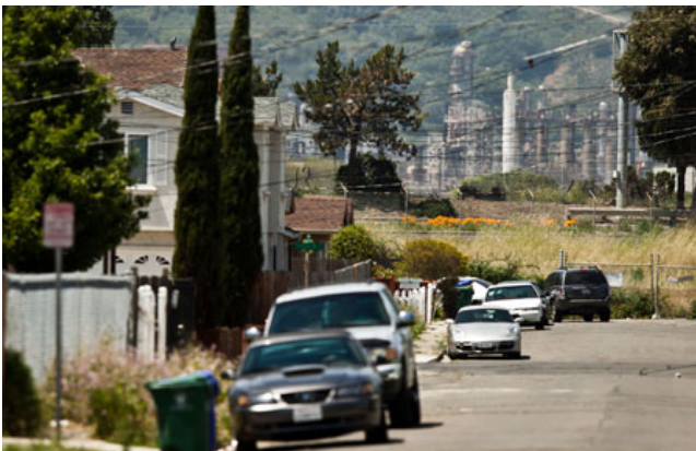
The Chevron petroleum processing plant is next to a residential street in North Richmond.
